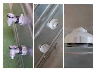
Make sure the rubber seal is on the inside of the tank
